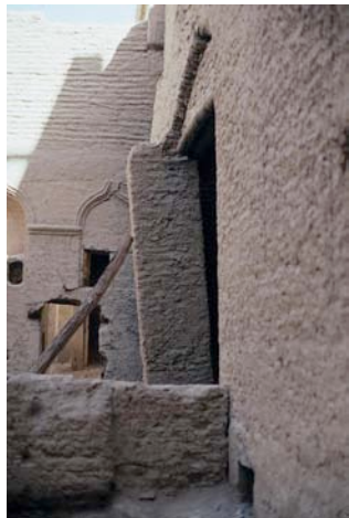
Fig. 31: The out-of-alignment pier supporting Dar Darwil's camel ramp is in critical condition.
