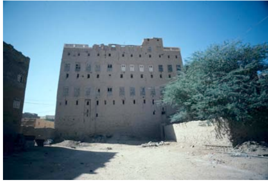
Fig. 105: Ba Heta had its two upper stories removed and is in fair-to-poor condition.
