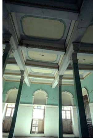
Fig. 50: Ceilings are highly ornate in al-Fijr. Note the cracks in the beams caused by structural damage in the room below.
