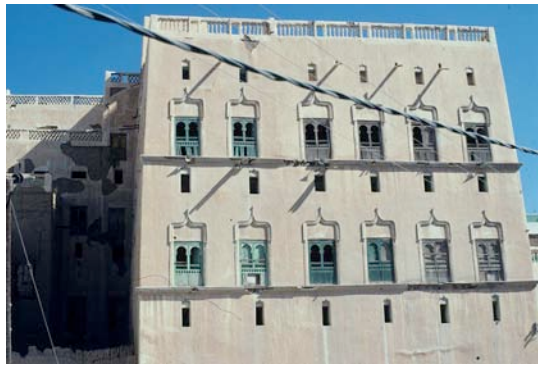
Fig. 89: Although rented, Dar Muhdar is in fair-to-poor condition. The west elevation faces the potter's square in the Sahil quarter.
