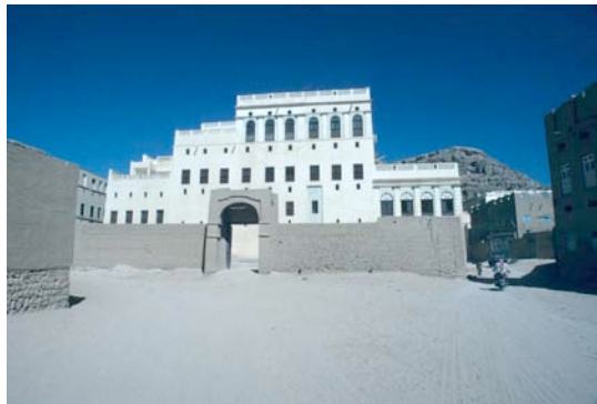
Fig. 103: Bayt Salih al-Tas al-Kaf is in excellent condition and still occupied by the son of the original owner.
