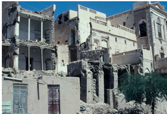
Fig. 59: The southwest corner of Bayt Abd al-Rahman bin Sheikh al-Kaf has partially collapsed.
