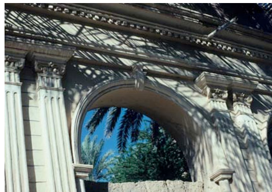
Fig. 92: Bir Yimani's exterior details indicate that the building may have been designed by Alawi Abu Bakr al-Kaf.
