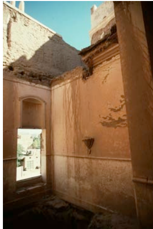
Fig. 29: The collapsed northwest wing of Dar Dawil, the oldest building of the 'Ishshah complex.
