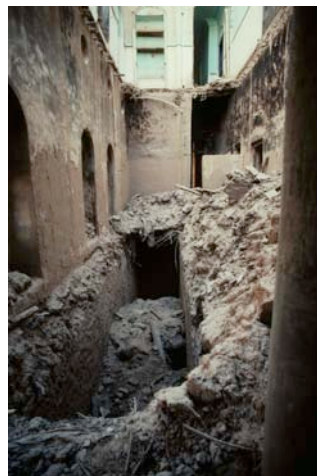
Fig. 28: The northwest kitchen wing of the 'Ishshah collapsed in 2001.
