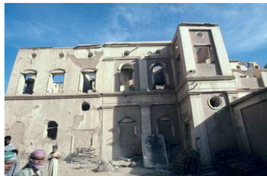
Fig. 12: The al-Kaf hospital was abandoned in 1975 when a new concrete hospital was built.
