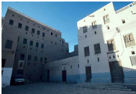
Fig. 119: Bayt Mugam al-Haddad is comprised of two structures, the newer of which is in excellent condition (at right). The earlier structure is in good-to-fair condition.
