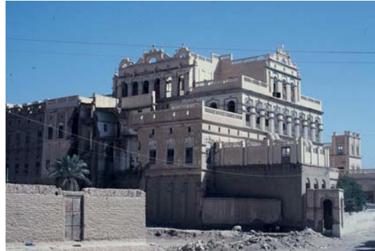
Fig. 26: A major collapse of the 'Ishshah's west elevation load-bearing wall occurred in 2000.
