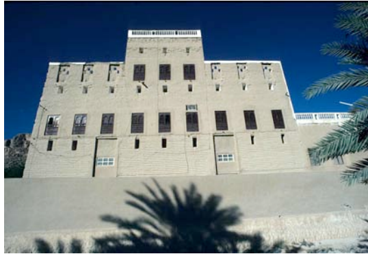
Fig. 117: Bayt Mahsun al-Hadi is in excellent condition.
