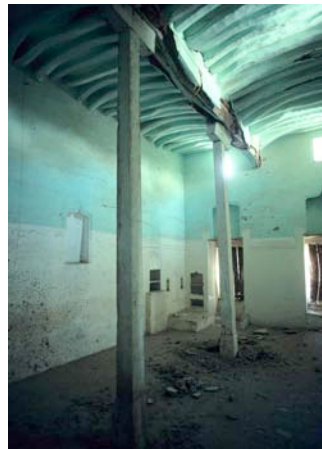
Fig. 52: A beam in al-Fijr with termite damage that needs to be shored immediately. Emergency funds have been requested from the SFD.
