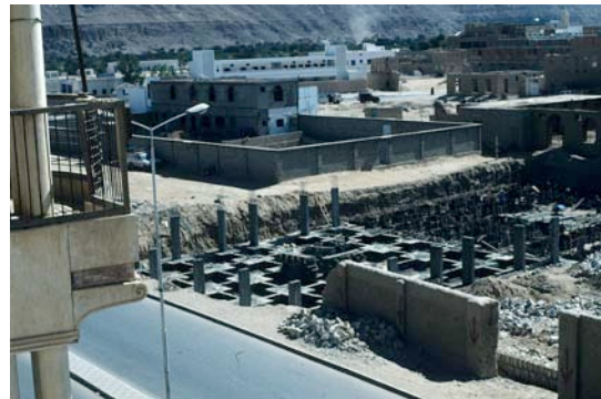
Fig. 8: New concrete construction is in progress across the street from Dar al-Salam in the historic core of Tarim.
