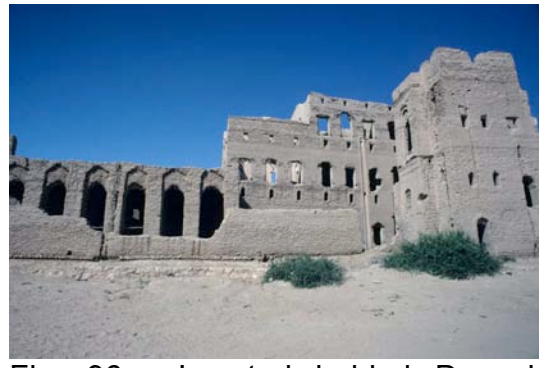
Fig. 96: Located behind Dar al-Salam, Ba Hussain is in ruinous condition beyond repair.
