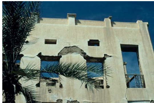
Fig. 76: Identified in 1999 as being in ruinous condition beyond repair, Lubnan was most likely designed by Alawi Abu Bakr al-Kaf.
