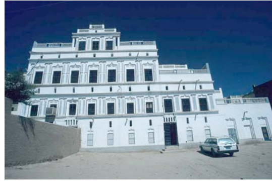
Fig. 106: Bayt Mayshur bin Hasan bin Sheikh al-Kaf is in excellent condition.
