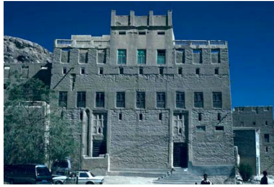
Fig. 114: Bayt Ahmad bin Abdallah bin Aidarus bil-Faqih is in good-to-fair condition.
