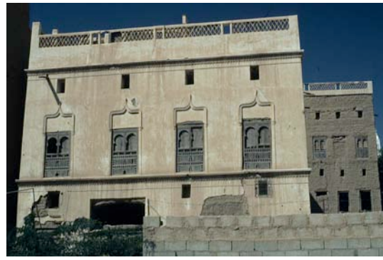
Fig. 68: The east elevation of al-Shatry is in good-to-fair condition.
