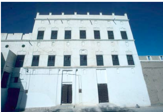
Fig. 87: Al-Madah's circular windows date it to the late nineteenth century. It is in good condition.
