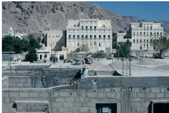
Fig. 7: New concrete buildings are being erected in the historic core of Tarim. This example is behind al-Fijr. The Aydid and Salmanah mansions are seen in the distance.
