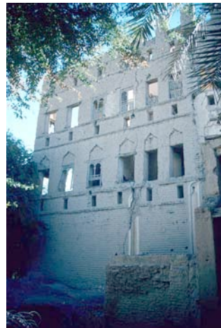
Fig. 72: Al-Mudarrabah, the country estate of 'Umar bin Sheikh al-Kaf, is in ruinous condition beyond repair.
