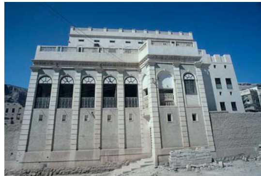
Fig. 104: The east elevation of Bayt Salih al-Tas al-Kaf is obviously a later addition.
