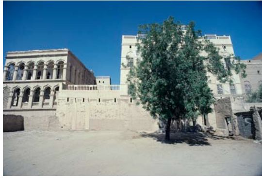
Fig. 81: Al-Majaff was identified as being in fair condition in 2000.
