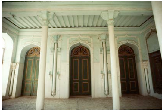
Fig. 19: The 'Ishshah boasts some of the finest examples of historic malas , a type of burnished lime plaster.
