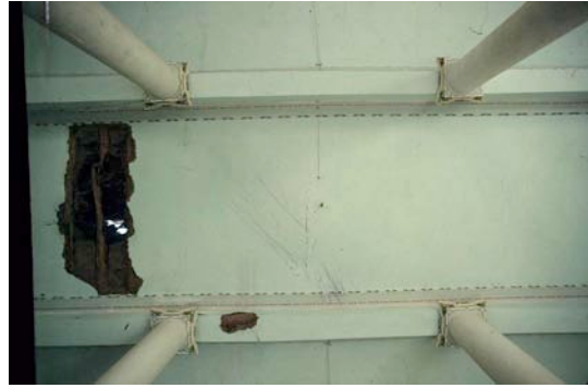
Fig. 38: The roofs of Dar al-Salam are in relatively good condition, although there was a hole in the roof over Room 133, that was repaired during documentation with Social Fund for Development (SFD) funds.
