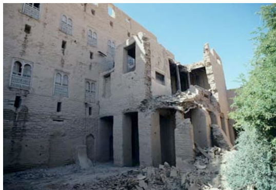
Fig. 43: The northwest kitchen wing of the Hamtut collapsed in 2002.
