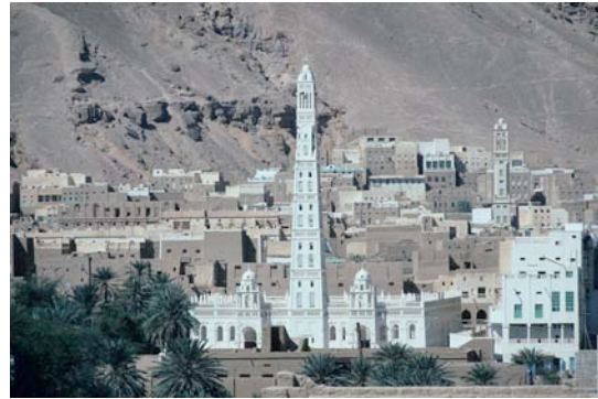
Fig. 6: Tarim's al-Mihdhar Mosque's minaret is constructed of unreinforced mudbrick and, at forty-one meters, is the tallest minaret on the Arabian Peninsula.
