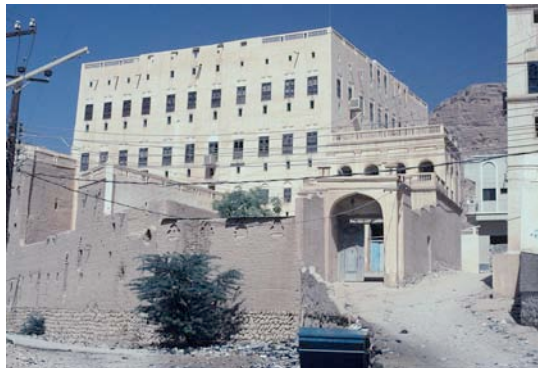
Fig. 95: Bayt Salim Abu Bakr al-Kaf is also located in the Sahil quarter on the potter's square and is in good condition.
