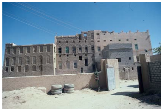
Fig. 100: Bayt Salih bin Ahmad al-Kaf is in good-to-fair condition, with some repairs ongoing.
