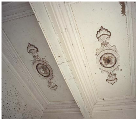
Fig. 91: A ceiling from the interior of Bir Yimani shows the mansion had a rich decorative scheme.
