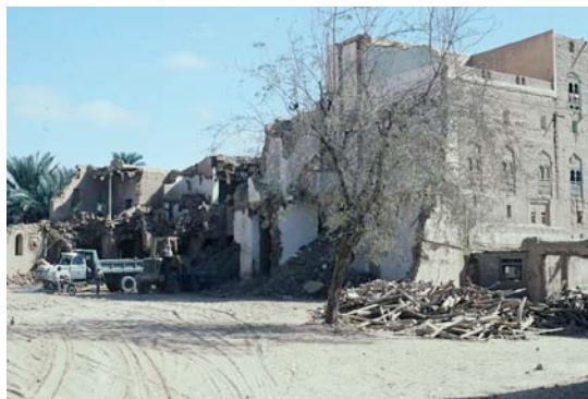
Fig. 83: Al-Majaff has been partially demolished and the site prepared for new concrete construction.
