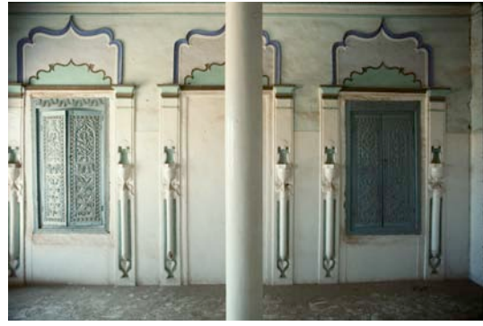
Fig. 18: Built-in closets in the 1920s 'Ishshah have elaborately carved wood doors.
