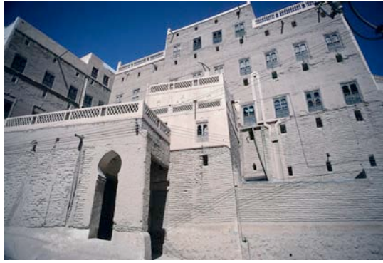
Fig. 93: Bayt Ahmad bin Ali al-Kaf is still occupied by the original family and is in good-to-fair condition. It is located in the Sahil quarter.
