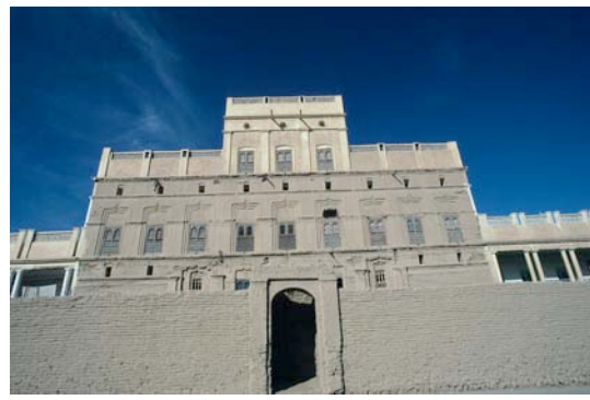
Fig. 108: Bayt Hussain bin Ahmad al-Kaf is near al-Mihdhar mosque and is in good-to-fair condition.
