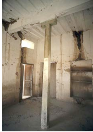
Fig. 45: The rooms in the northwest corner of al-Ryad are in danger of collapse. Emergency stabilization funds have been requested from the SFD to repair roofs.
