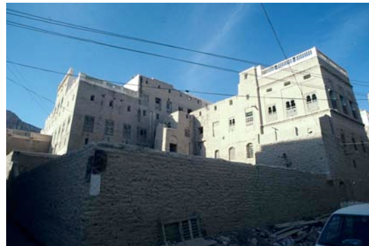
Fig. 80: Al-Nuwaydara consists of two buildings and is in good condition.
