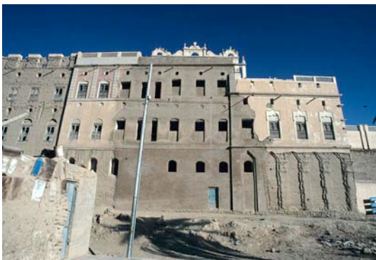
Fig. 27: The west elevation of the 'Ishshah was rebuilt in 2003 under the direction of master mason Karami Faraj al-Tamur.
