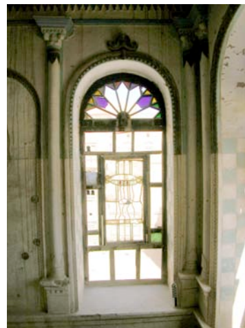
Fig. 16: Most of the 'Ishshah's Art Nouveau stained glass is in poor condition.
