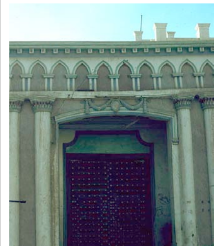
Fig. 121: Al-Ranad currently functions as the police station and post office. It requires restoration.
