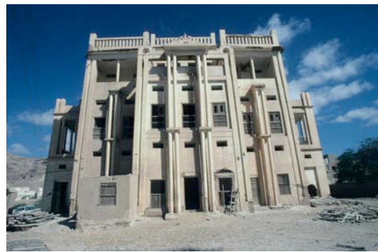
Fig. 44: Another Art Deco villa designed by Alawi Abu Bakr al-Kaf, al-Riyad is being proposed for reuse as the Museum of the Environment of the Wadi.
