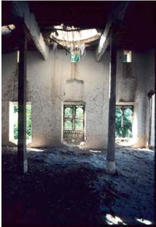
Fig. 73: The interiors of al-Mudarrabah are witness to its gradual demolition.
