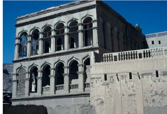
Fig. 82: Al-Majaff was noted for its Mughal-style pavilion which suffered partial collapse in 2002.
