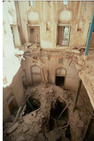
Fig. 30: The northeast wing of Dar Dawil has also collapsed.
