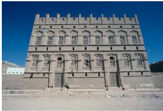
Fig. 47: The south elevation of al-Fijr, the mansion of the architect Alawi Abu Bakr al-Kaf. Adjacent to the Hamtut, it is being proposed for reuse as al-Awqaf Manuscript Library.
