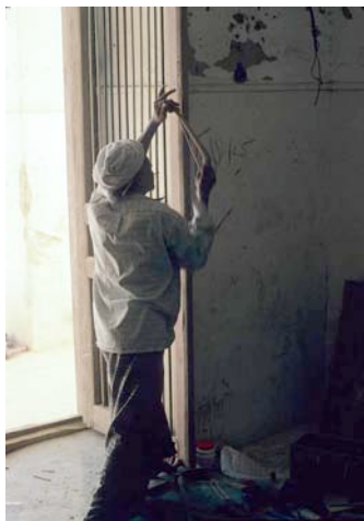
Fig. 39: Carpenter Salim Ba Hashwan restored Dar al-Salam's front door.
