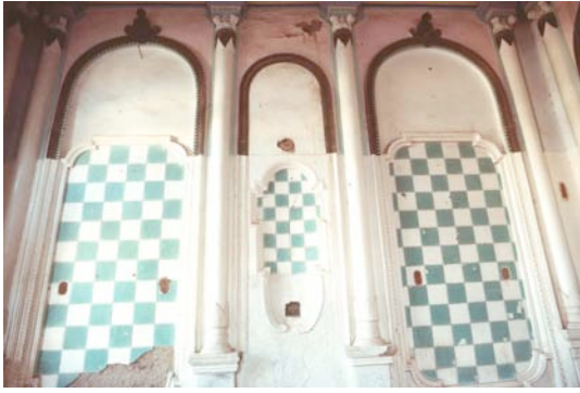
Fig. 25: The bathroom from the 'Ishshah's 1930s Baroque addition is a wonderful example of historic malas .
