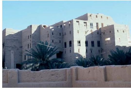
Fig. 66: Bayt Hasan Abdallah al-Haddad is abandoned, but in good-to-fair condition.
