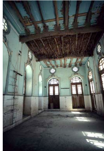
Fig. 58: The interior of Bayt Abd al-Rahman bin Sheikh al-Kaf has suffered from termite damage.
