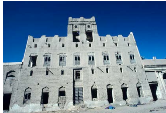
Fig. 90: Bir Yimani, the country estate of Muhdar bin Alawi al-Kaf, is in ruinous condition beyond repair.
