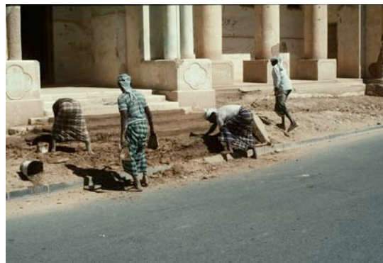
Fig. 40: Master mason Ghamdan Karama Ba Haji directed the repair of the front steps of Dar al-Salam.
